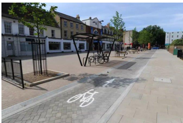
Image 5: Cycle lane in Lower Bridge Street.
